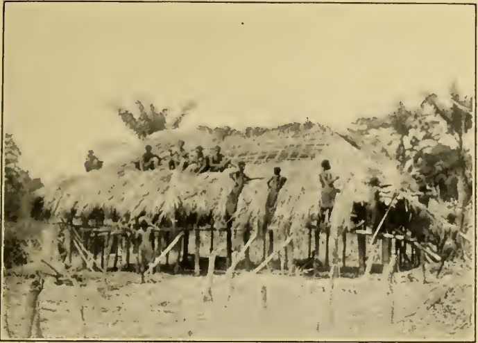
PUTTING THATCH ROOF ON THE CHAPEL Vanga
